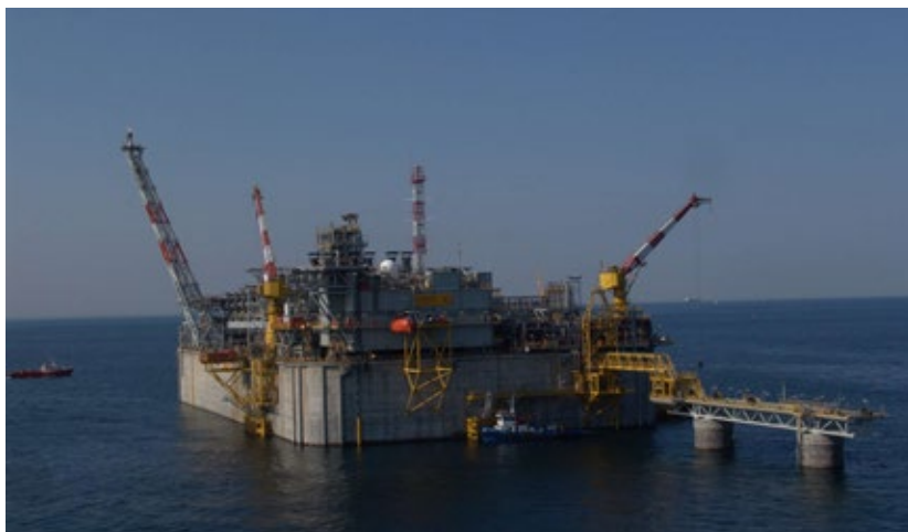
The Rovigo LNG terminal in the Adriatic Sea. (Edison)
